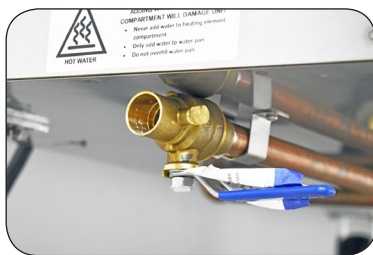
Detail View of Well Drain Valve located on the outside bottom of unit.
